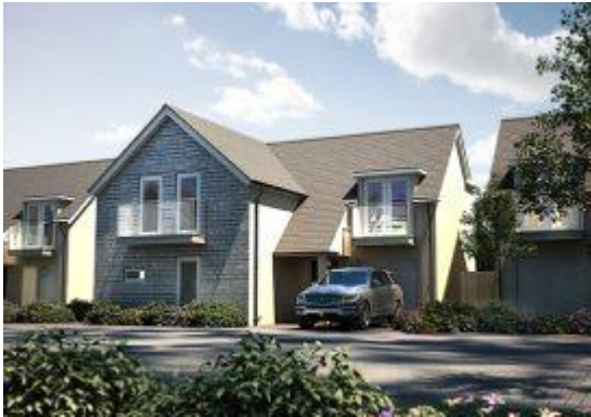
Bloor Homes have started work on the delivery of new homes at the former Pontin's Holiday Park in Brixham.
